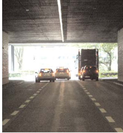
Overexposed image with view outside tunnel not clearly visible.
