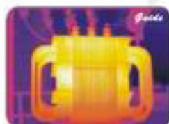
Inspect electricity hot point
