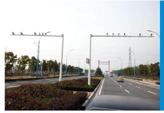
CP200 Automatic Number Plate Recognition system is mainly used to record image of each vehicle at the entry/exit of road and important road section. The license plate number will be recognized automatically. By analyzing the vehicle license plate, it can capture the blacklist vehicle and count the traffic flow. This system can do great help to seek suspect and improve the traffic efficiency.
